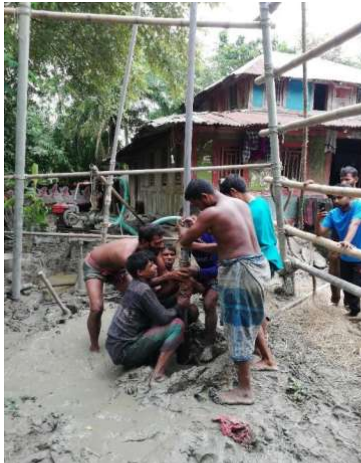
Figure 2-4: Installation of Monitoring Well
