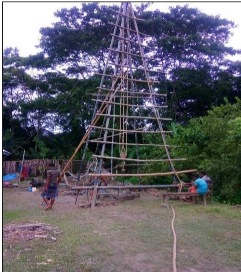
Figure 2-3: Drilling Procedure of Monitoring well.
